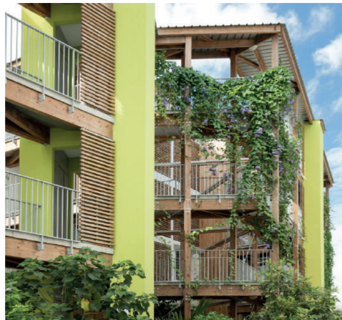
© Co-Architectes, Les Mahots
