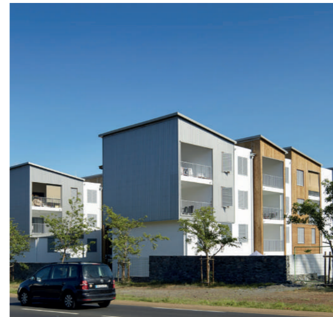
© Co-Architectes, Les Mahots
