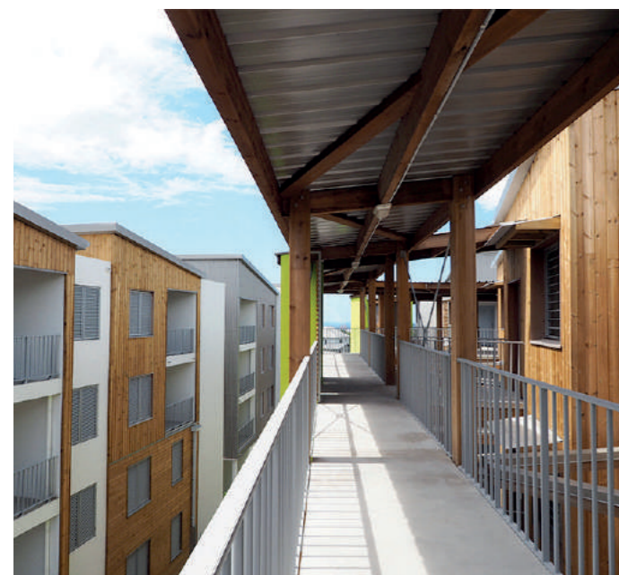
© Co-Architectes, Les Mahots
